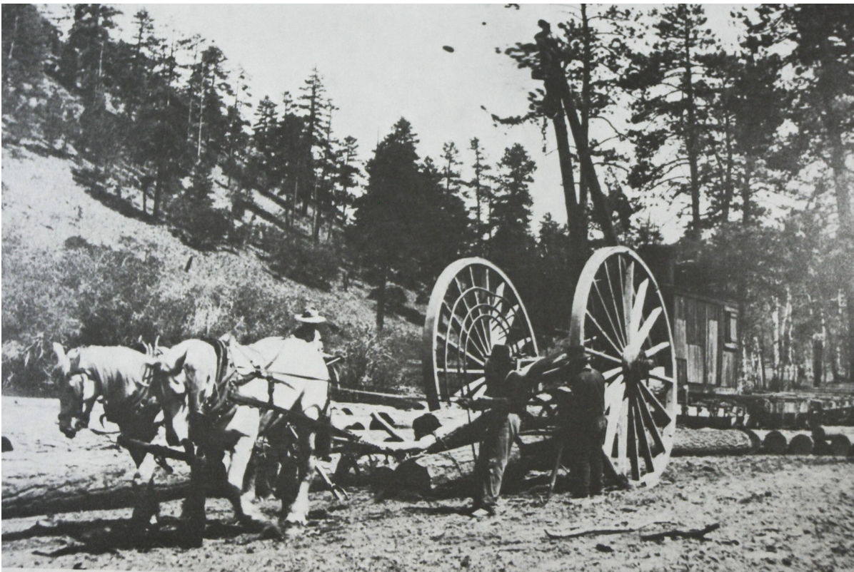
Moving Logs: The logs are chained beneath the axle
