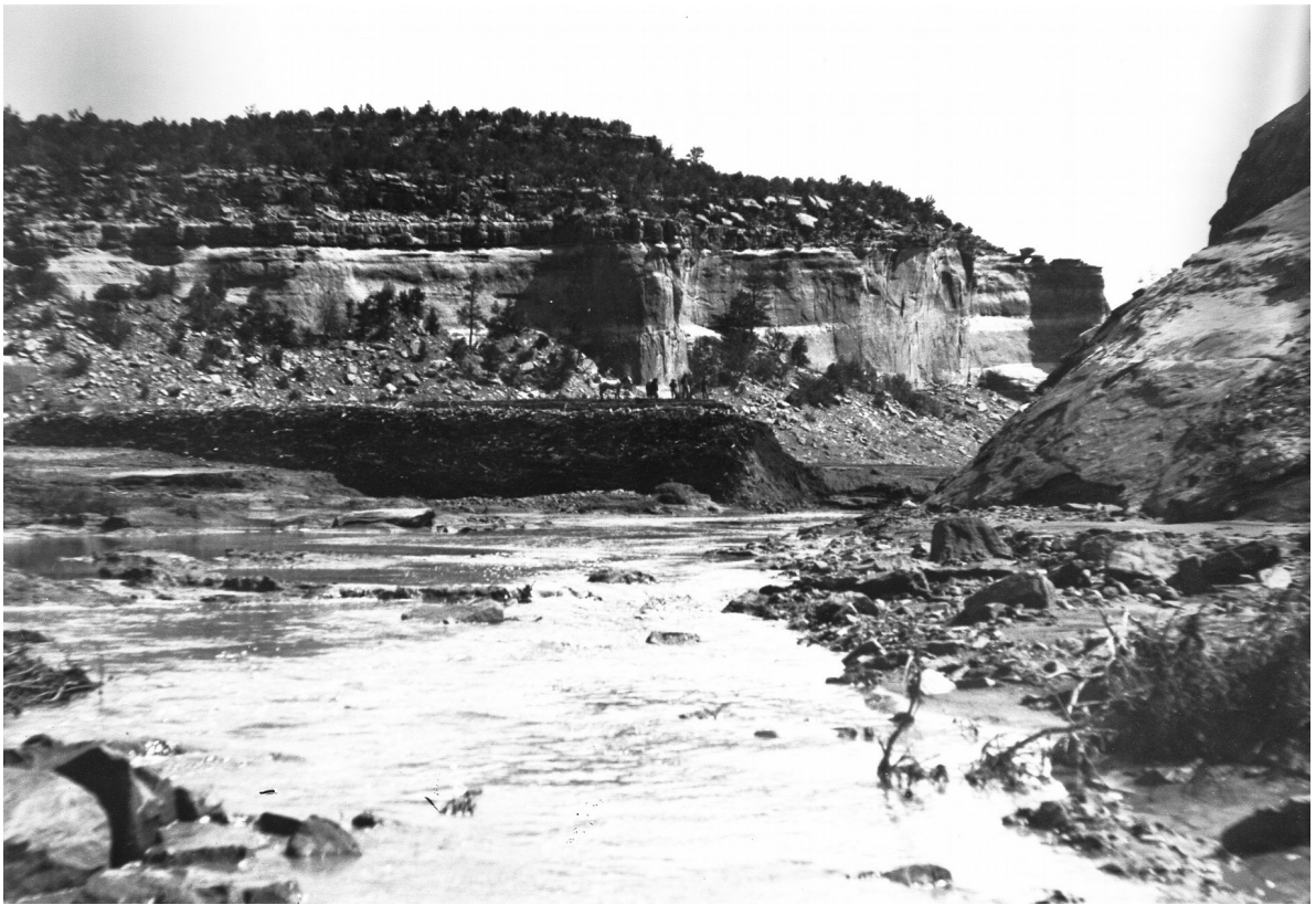
Ramah Dam Washes Out 1897
