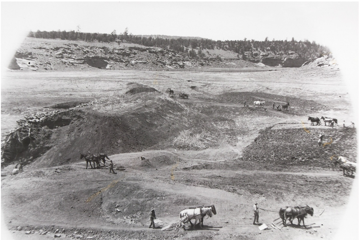
Ramah Dam Being Repaired
