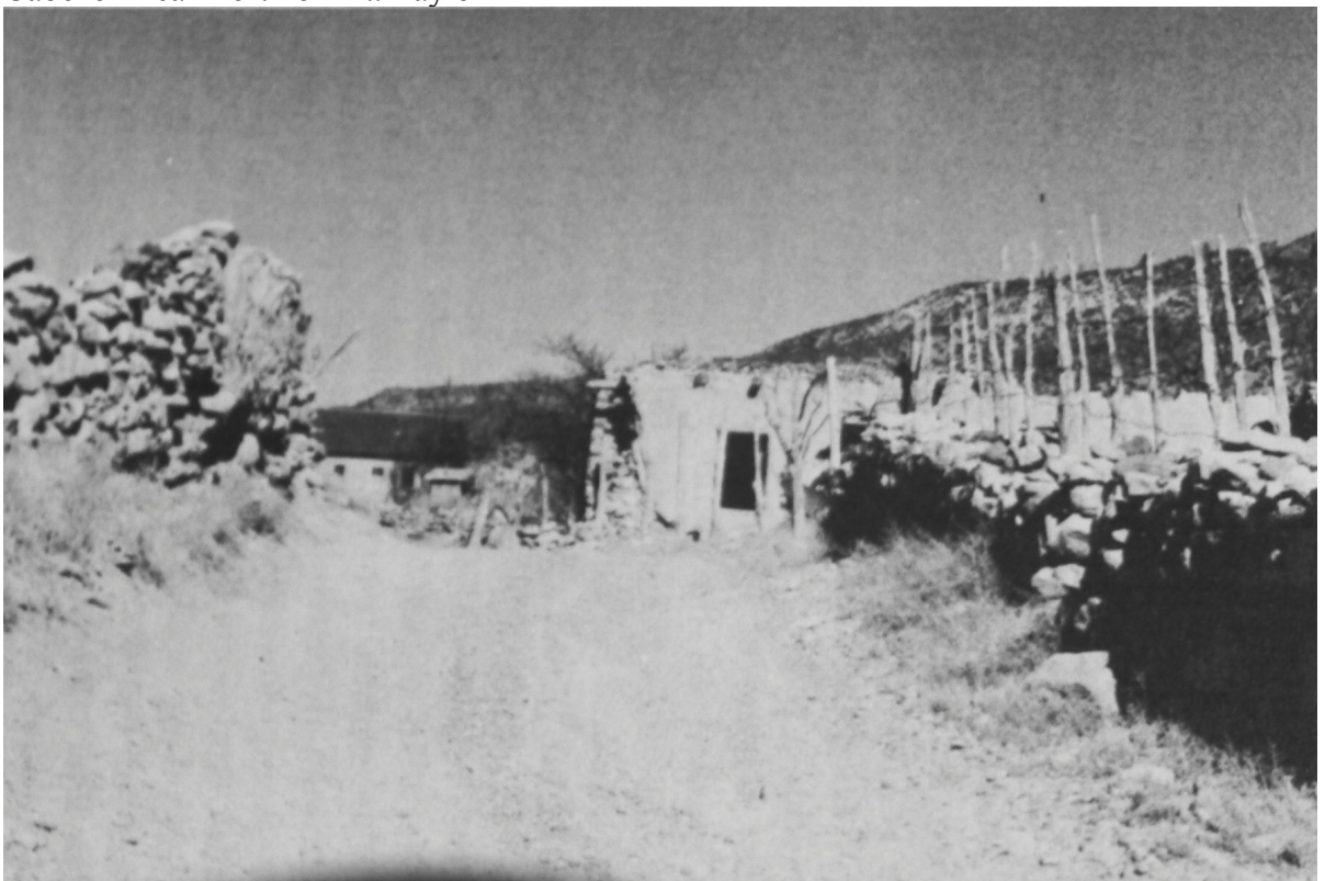
Street in Cebolleta with walls of old fort
