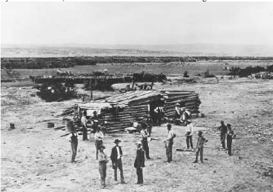
Grant's Camp, Railroad Construction
